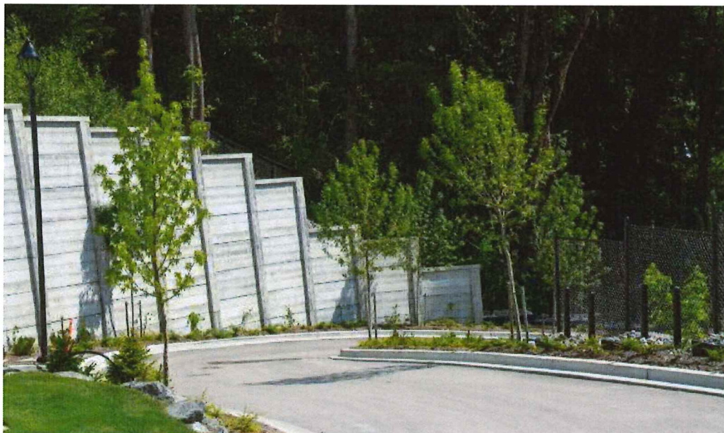
Typical Anchor Fast Retaining Wall
