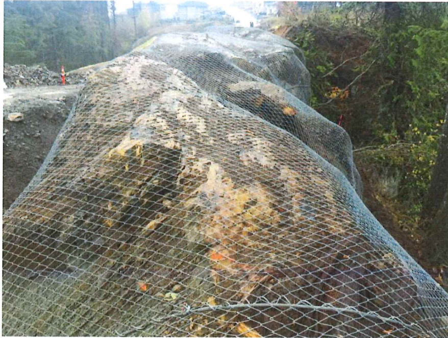
Wire Mesh Pinned to Rock Face
