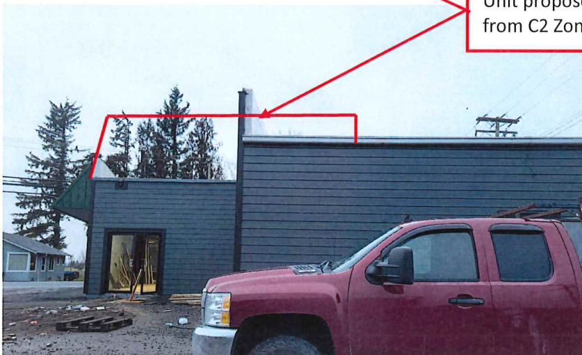
Building Face - South
