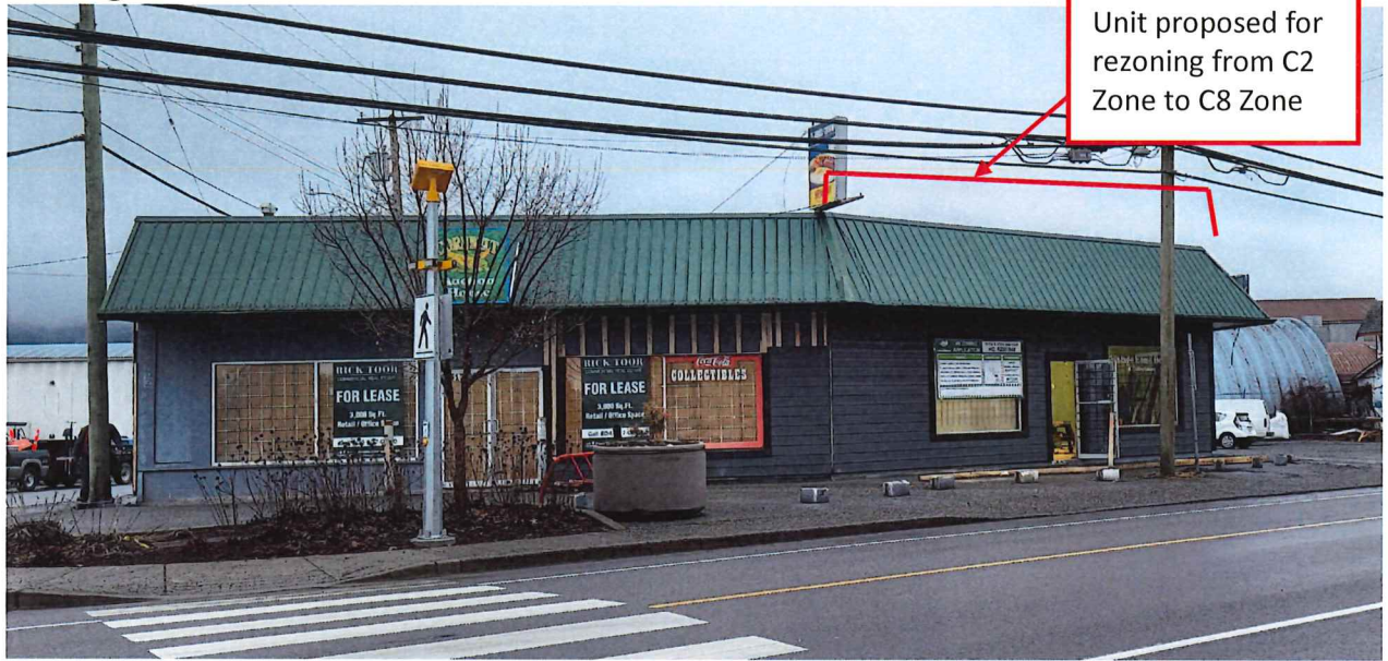
Building Face - North
