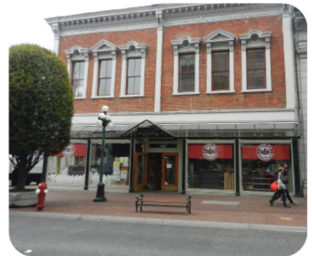
Photo 3 - Views from inside the store can help promote safety on the street
