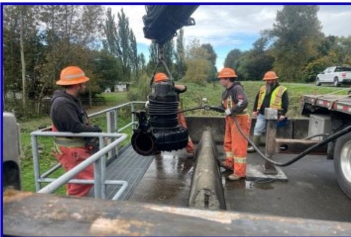
Pumps being lowered into the water
